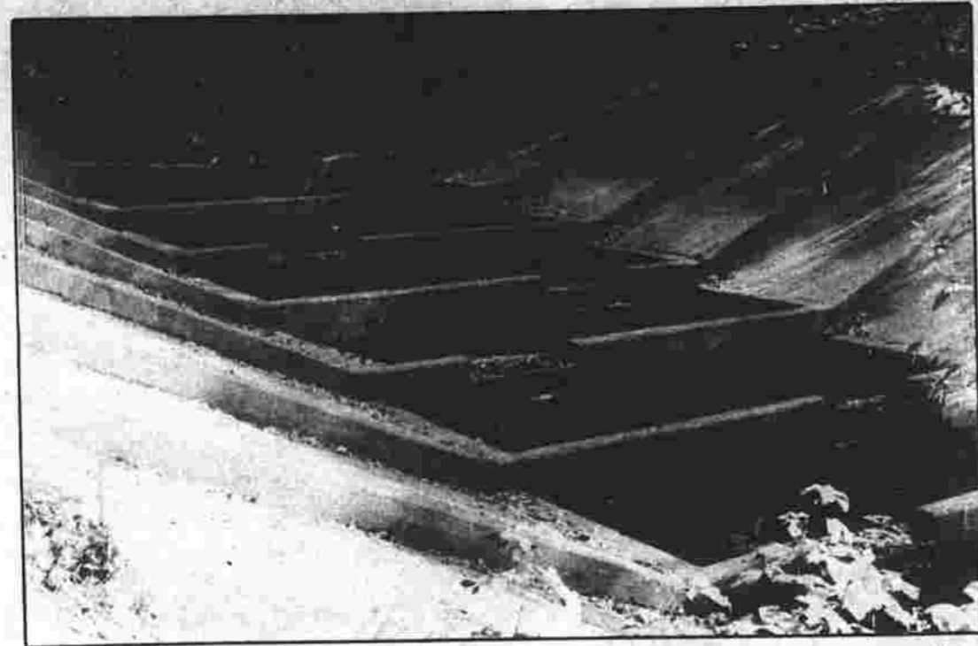
Fish Ladder at Charter Oak Park Herald Photo by Pinto
